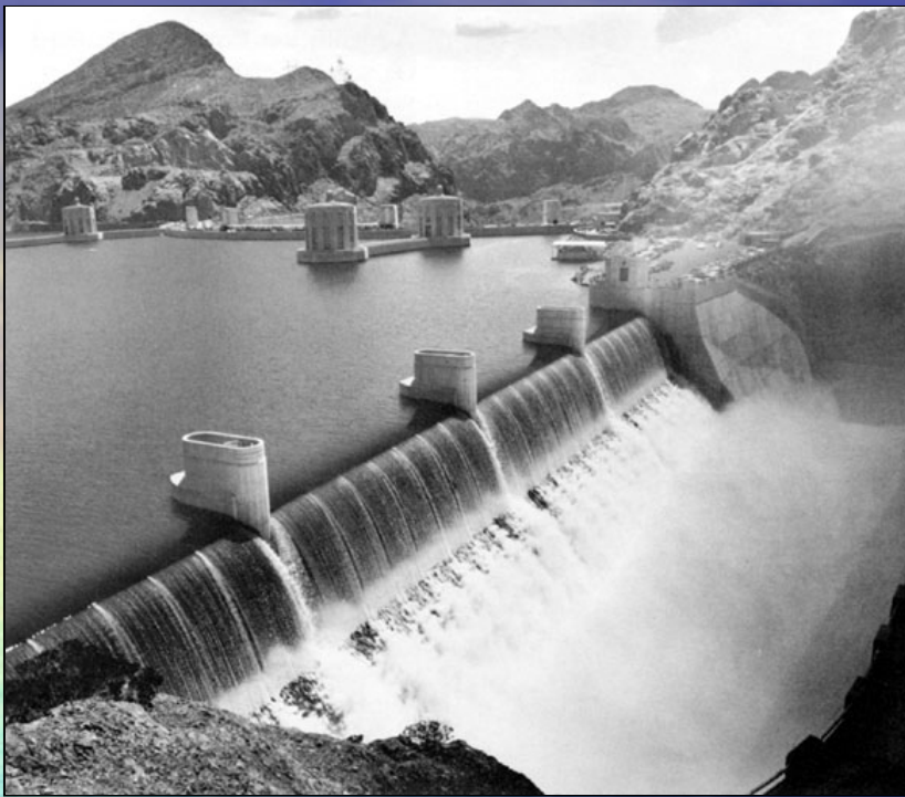
Spillway test August-October 1941
