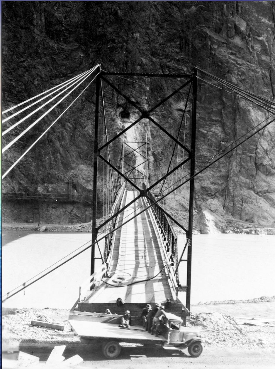
Wire suspension bridge serving the construction adit (dark hole in background) for the Arizona diversion tunnels.
