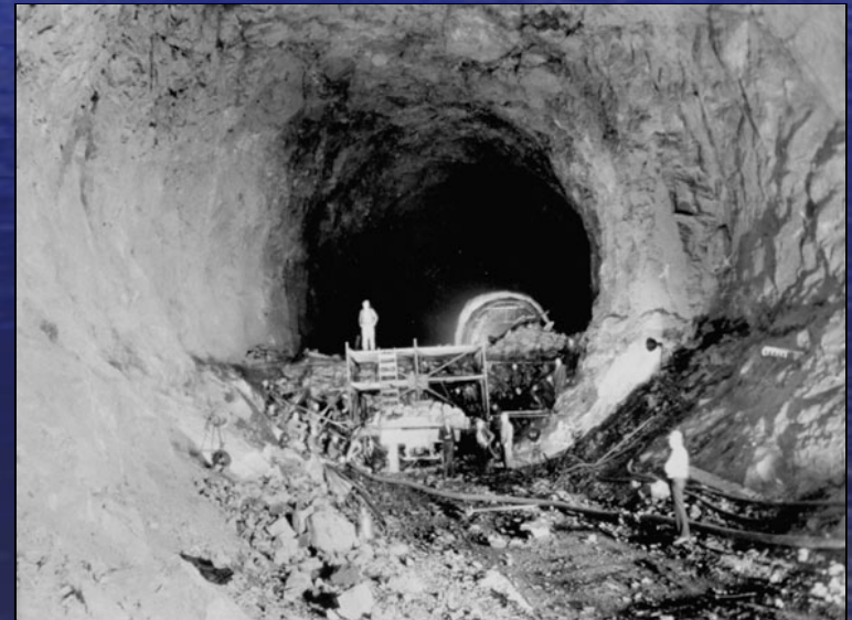
Ready for lining
