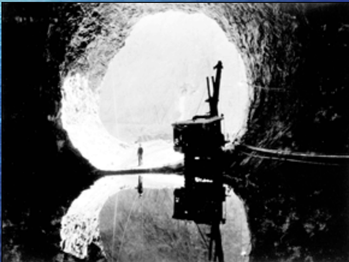
Finished 56 foot diameter bore
