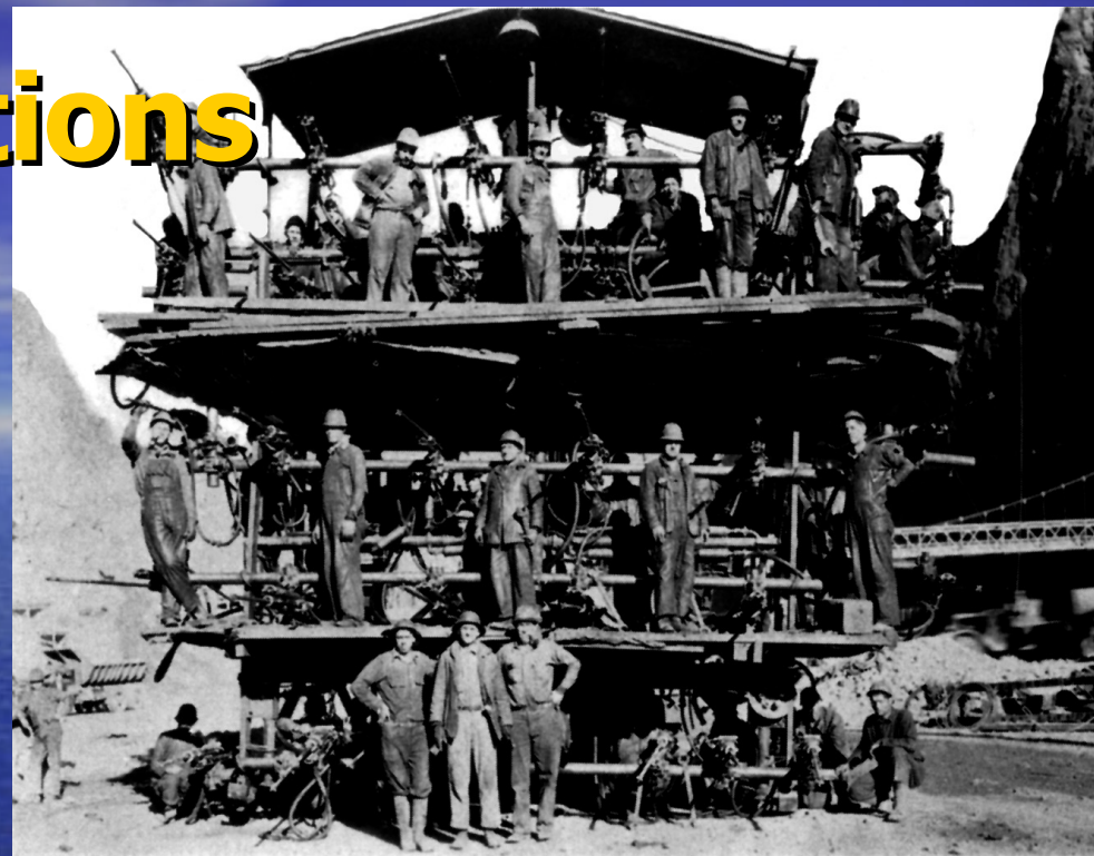
World's first drilling jumbo
